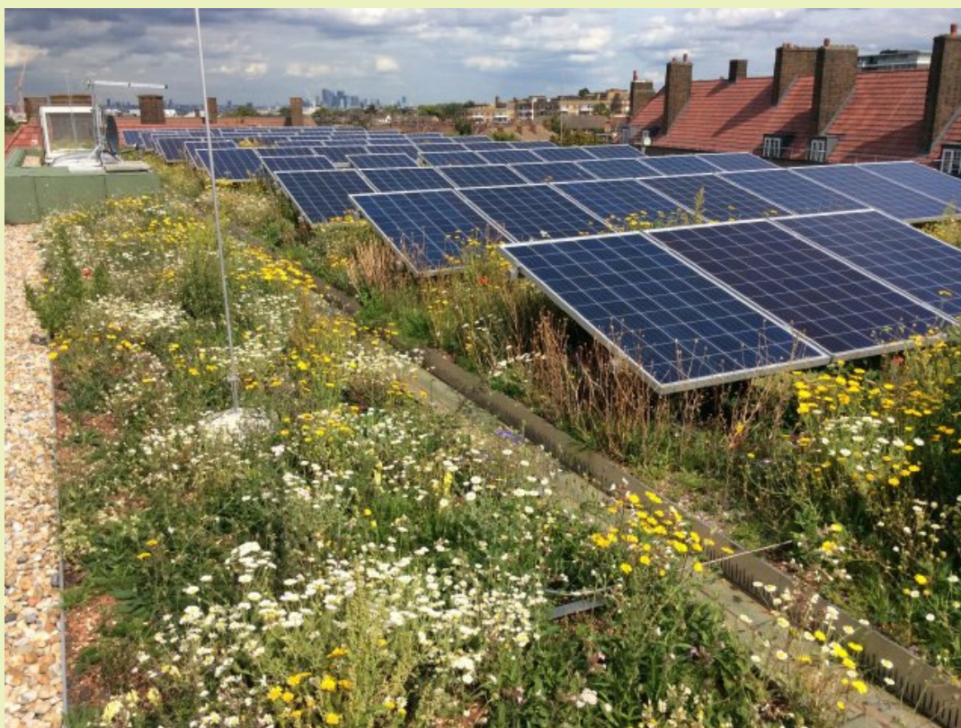
An example of a biosolar roof. Greening and solar panel provision for heating and hot water can be co-located on roofspace.
